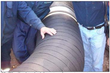
**SP-6<sup>TM</sup>** will reduce the deformation of corrosion coating systems caused by soil stress. It acts as a slip plane to relieve soil stress.
