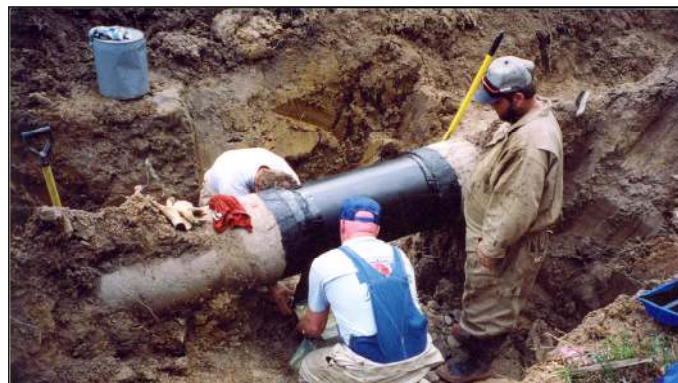
606 Filler Compound filling irregular transition areas.
