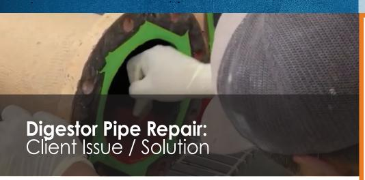
A Wastewater Treatment Facility was experiencing significant issues with digestor pipes clogging and needed some digestor pipe repairs and upgrades. Over time, an 8-inch diameter pipe had become choked down to a 1-inch diameter due to buildup on the pipe walls. This buildup caused back pressure issues and placed a strain on the pumps.
