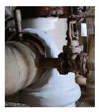
Resimac Resimetal 108 Pipe Repair Tape is a high performance rapid curing moisture activated repair bandage specifically developed for the repair of leaking pipes. 108 Pipe Repair Tape is ideal for systems
