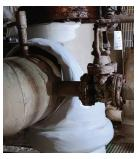
**Resimac Resimetal 108 Pipe Repair** Tape is a high performance rapid curing moisture activated repair bandage specifically developed for the repair of leaking pipes. 108 Pipe Repair Tape is ideal for systems
