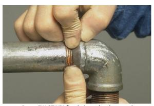
5. Press FIX STIX™ firmly into the damaged area to ensure a solid fill.
