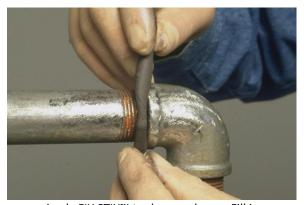
Apply FIX STIX™ to damaged area. Fill in holes, cracks or offsets.
