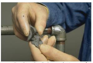
Knead together the inner and outer core of
