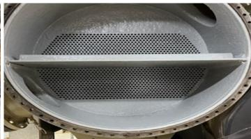
Our client had existing chillers that had never been coated before. Upon inspection they noticed a lot of galvanic corrosion on the tube face sheet and lid of the chiller.
