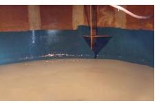
This was a 30 year old fiberglass tank that had many leaks and would not hold pressure. We specified ResiMetal 106XF for the holes and to line the entire bottom and ResiMetal 209 EIP PU three feet up the side to assure integrity. We also provide the value added service of technical supervision. **Call us to find an approved USI installer - 248.735.7000!**
