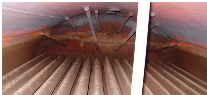
The waterside of a firetube boiler that was shut down and left full of water is shown. Brown areas show where the pipes and walls were covered with water. The orange line shows where corrosion has occurred above the water level because the boiler was not laid up with a vapor-phase corrosion inhibitor. | Photo credit: Cortec Corp.
