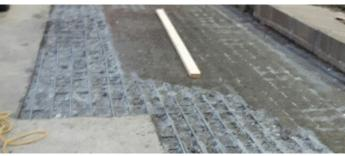
Epoxy resin based solvent free hig el screed. The product has been designed to be applied to uneven concrete surfaces to a wet film thickness of 10-30mm (3/8"- 1 1/4"). On curing the product will ensure any imperfections on the surface
