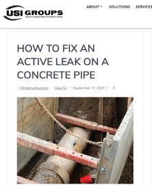
**STEP 1** – The pipe was first cleaned and prepped according to the Technical Data Sheets of the products to be used to create a long term solution.
