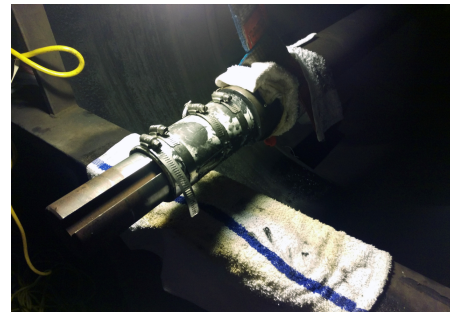
Hose clamps were then used to hold the PVC pipe and heat was applied to force cure
