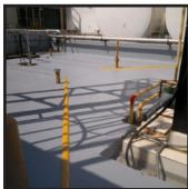
The USI Team prepped the area first and repaired many cracks. USI also added much needed burms to make over flow liquids drain in the correct direction. Products used were an Epoxy Concrete Repair, an Epoxy Sealer, an Epoxy Coating and an Epoxy Slip Deterrent.
