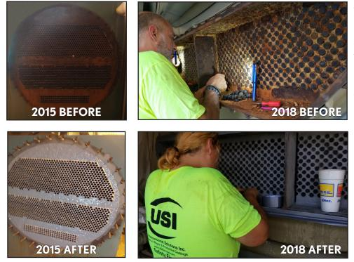
A Major Big Ten University was experiencing galvanic corrosion, also known as bimetal corrosion, which was eating away at the metals and causing tubes to plug. This Michigan University wanted to lower their energy cost and felt a hydrophobic ceramic enhanced polymer coating would provide a smoother surface and reduce energy bills. Having worked with the **USI Team** before, they called us in to work on this important project.
