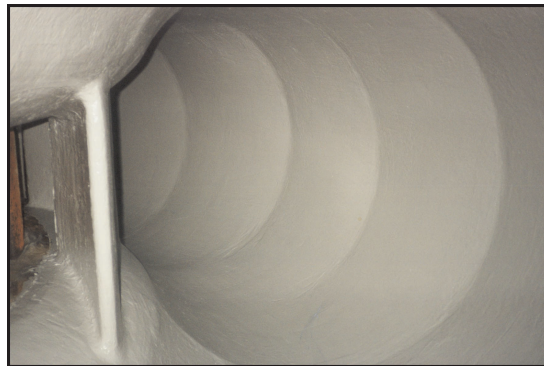
Scroll Case Lining at a Hydroelectric Powerplant
